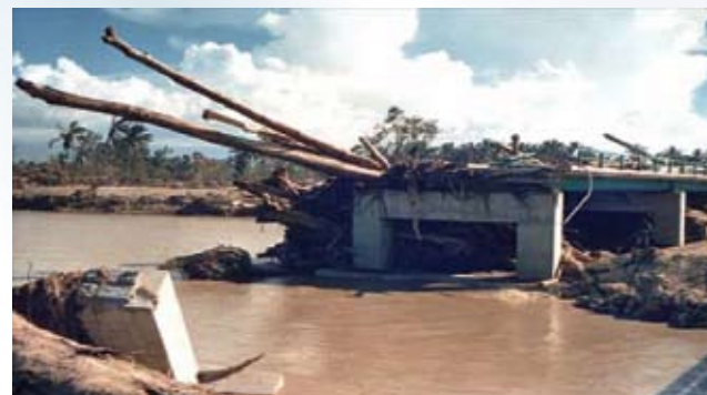
Figure 7 Smashed bridge over the Lungga River near the capital Honiara in Solomon Islands, shortly after a major flood in May 1986. The behaviour of island rivers remains poorly understood due to a lack of consistent hydrometric gauging and analysis.
