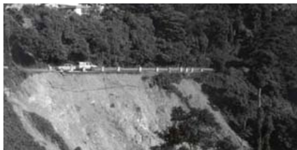
Figure 8 Shallow translational landslide in Suva city, the capital of Fiji, after prolonged wet weather in May 1997. Slides, debris flows, rockfalls and other types of landslides are responsible for many deaths on steep islands each year, but warning systems are non-existent or inadequate.
