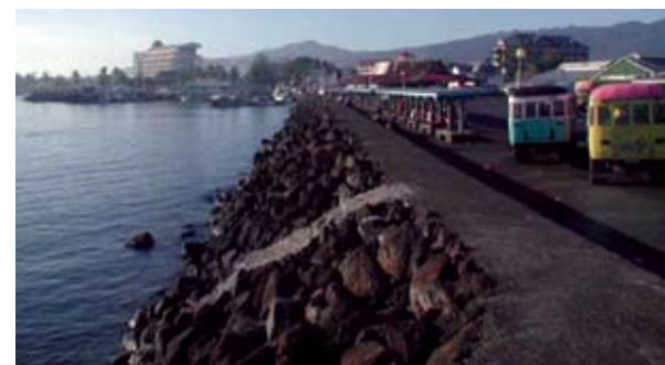
Figure 10 Modern seawall protecting Apia, the capital of Samoa. These kinds of seawalls are expensive to construct (from limited budgets) and are not appropriate for every type of island shoreline. Mangrove rehabilitation may be a cheaper option in the face of increased threats of sea-level rise.
